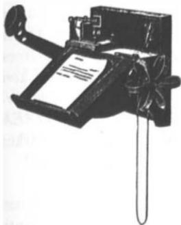
*A telephone set combining a small writing desk, an Edison transmitter, and a Phelps receiver.*
